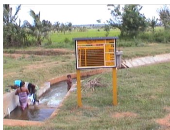
Name Boards fixed at the head of each Distributary Canals used to communicate the Water Budget of each DCFOs having about 300 Farmers having 1 Ha each
