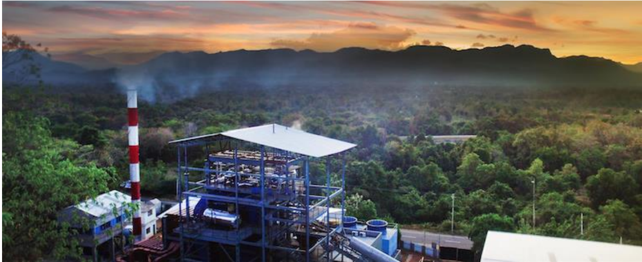
Loggal Oya Biomass Power Plant (2MW from 80 metric tons of fuel wood).
